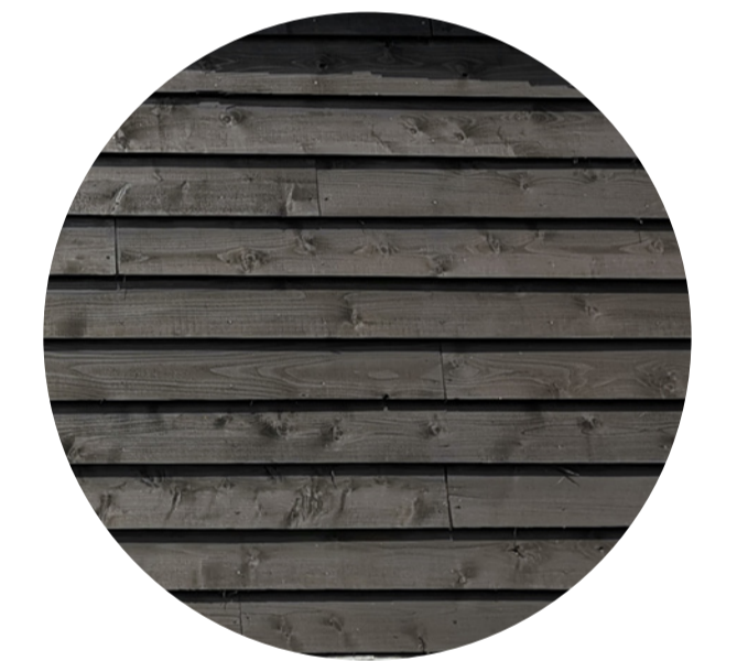
Painted / stained timber
